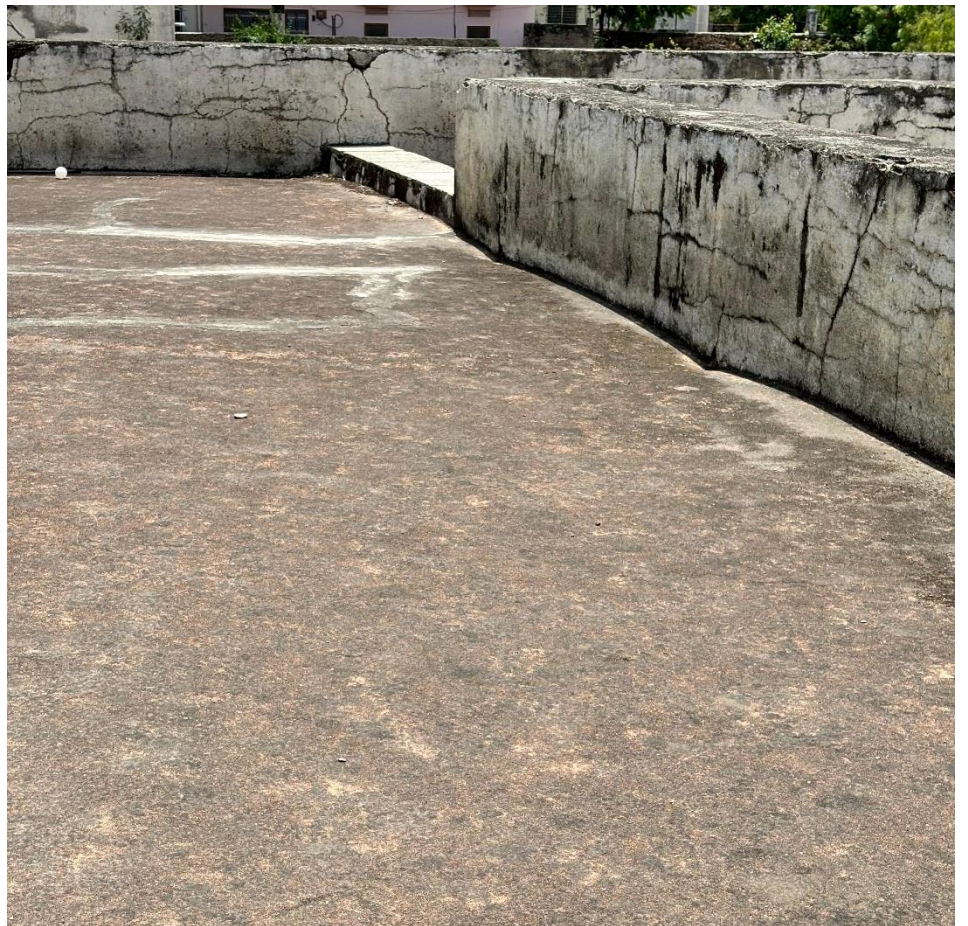
Lime Concrete roof top
