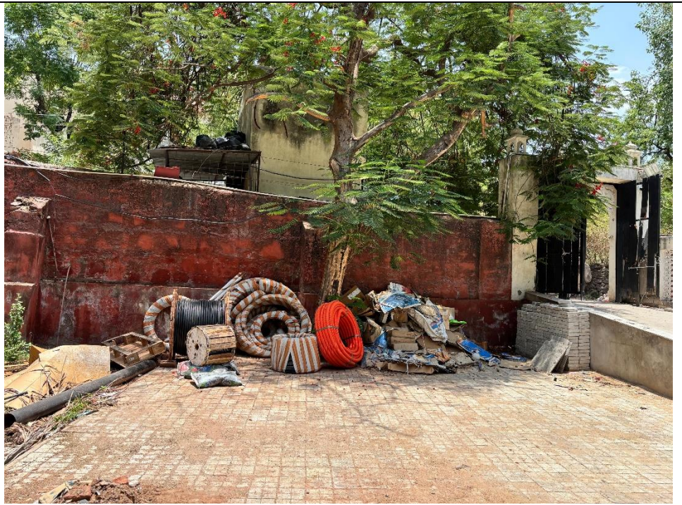
Entry gate wall to be de-plastered and lime plastered.
