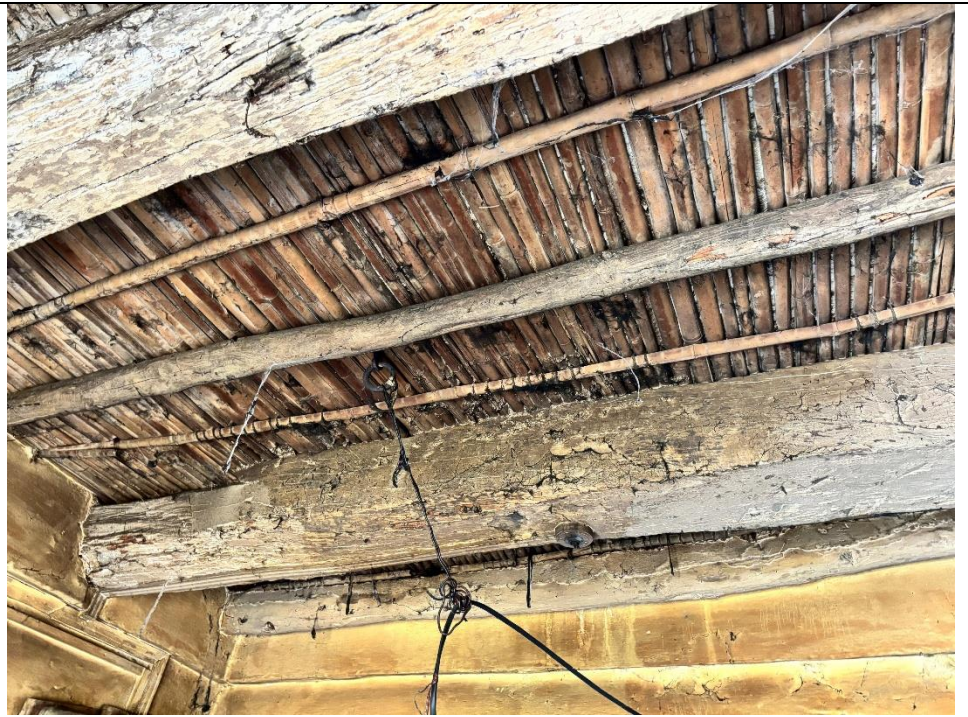
Wooden beam and bamboo stick reinforcement system roofing
