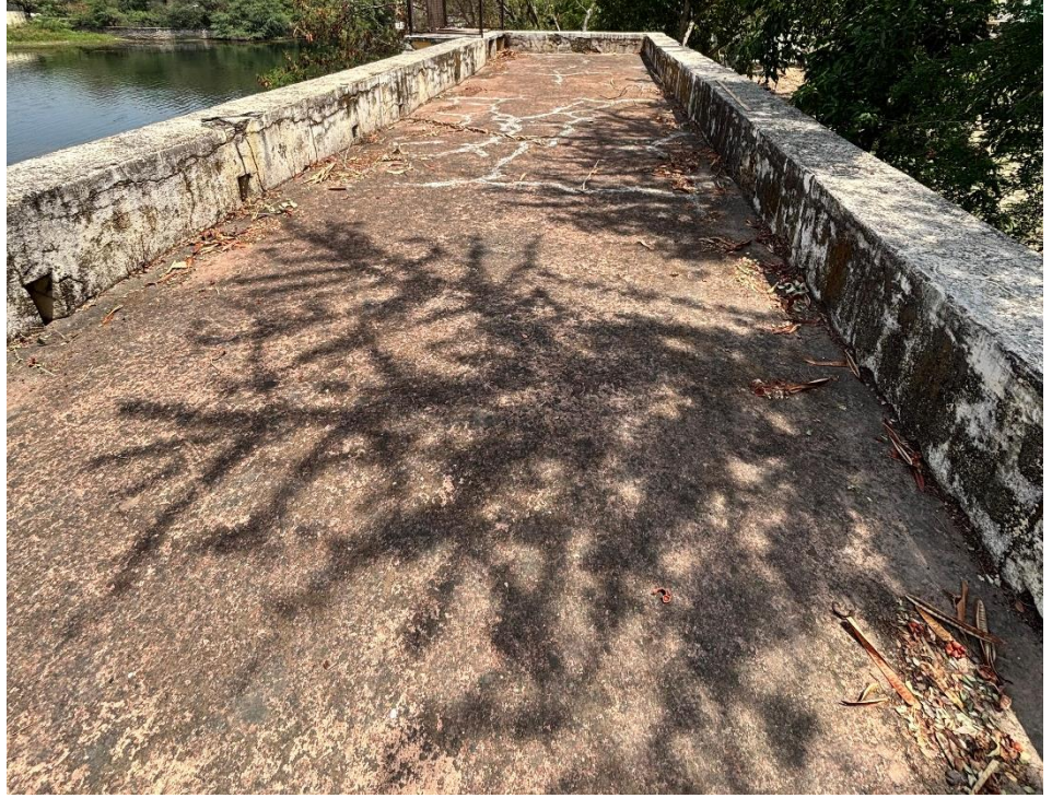
Roof top of the monuments in lime concreting
