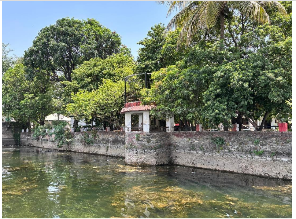
Retaining wall along the lake
